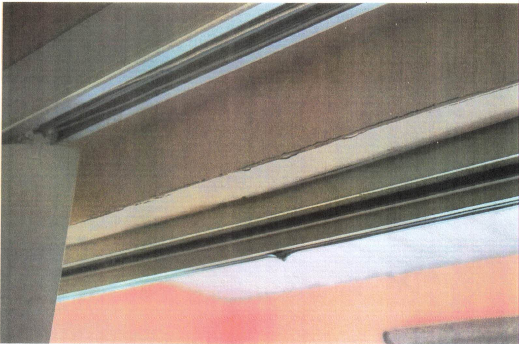
TYPICAL DRYWALL CRACKS – CONDO TO MONITOR FOR PROGRESSION - MAINTENANCE ISSUE
