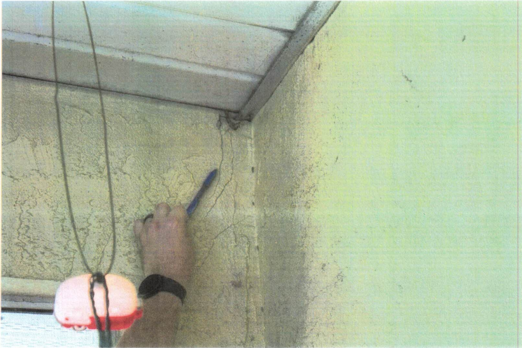
TYPICAL STUCCO CRACKS – CONDO TO MONITOR FOR PROGRESSION - MAINTENANCE ISSUE
